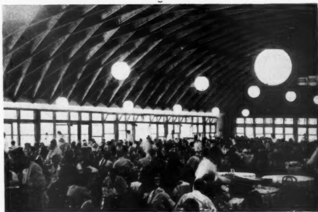
Three photographs of Unity House, the camp of the International Ladies' Garment Workers Union in Pennsylvania. This organization is one of the most energetically progressive in U.S.A. and Unity House has been largely reconstructed by William Lescaze. Top, dining hall and lounge; centre, the belvedere; right, the dining hall—showing the lamella roof construction.
