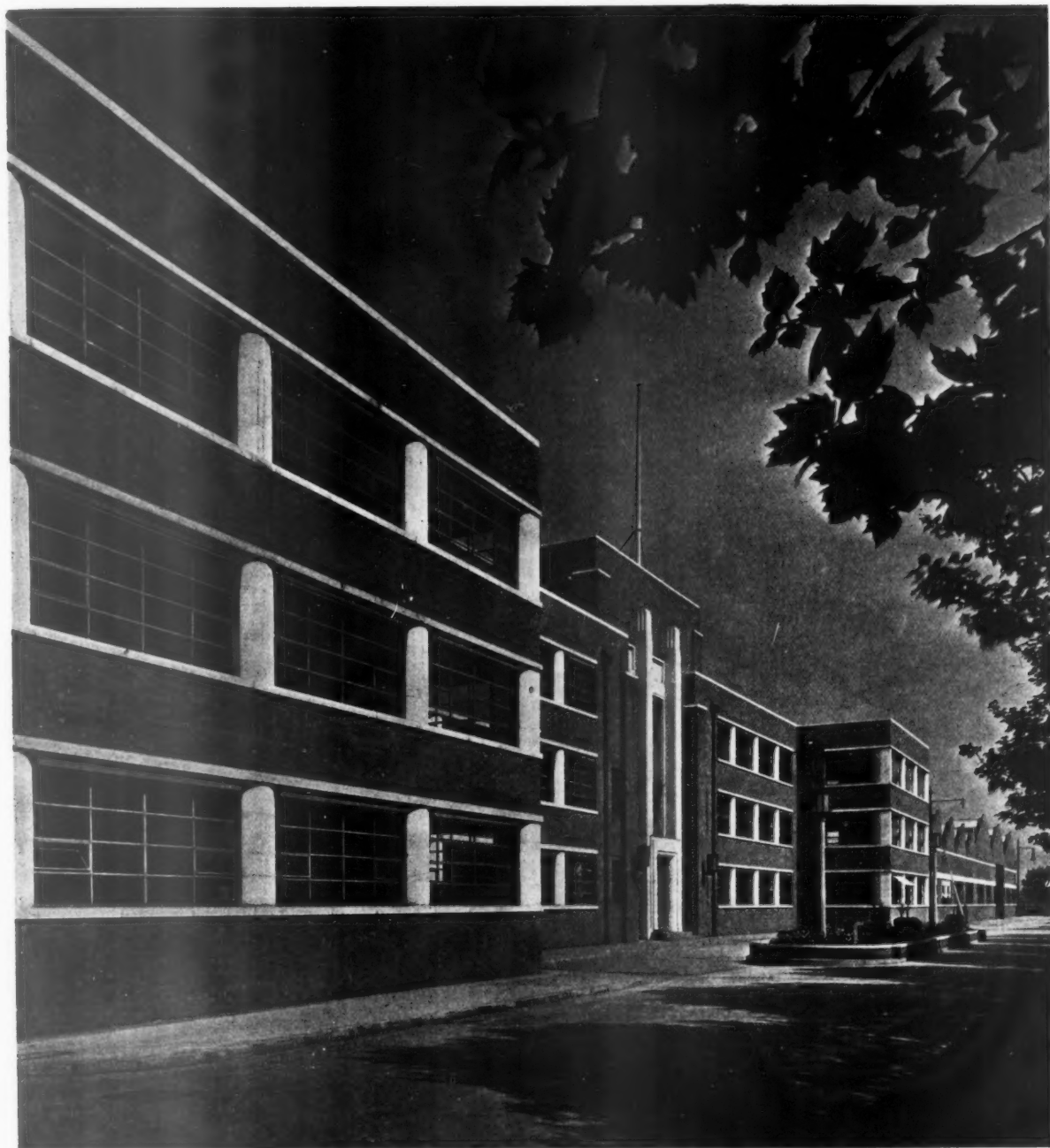
Factory at Ferry Lane, Tottenham, for Messrs. Keith Blackman. Architect : Clifford, Tee & Gale. Contractors : F. & H. F. Higgs Ltd., Herne Hill.
