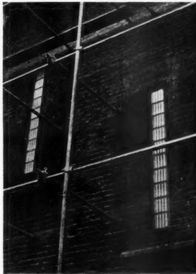
A method of protecting windows without excluding daylight at St. Stephen's (L.C.C.) Hospital, Fulham. The windows are partially bricked up, leaving a narrow vertical slit which is glazed with glass bricks. Right, an interior of a window on landing, using glass bricks.
