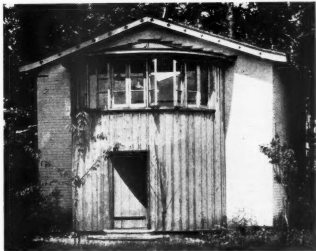
3 Windows, opening in and opening out, with external horizontal boarding and internal plaster.
