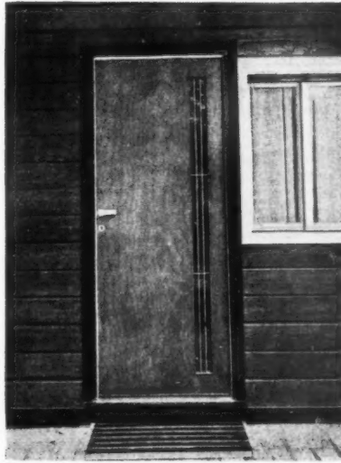
2 Projecting door frame with horizontal boarding. (E. Faludi, Italy.)
