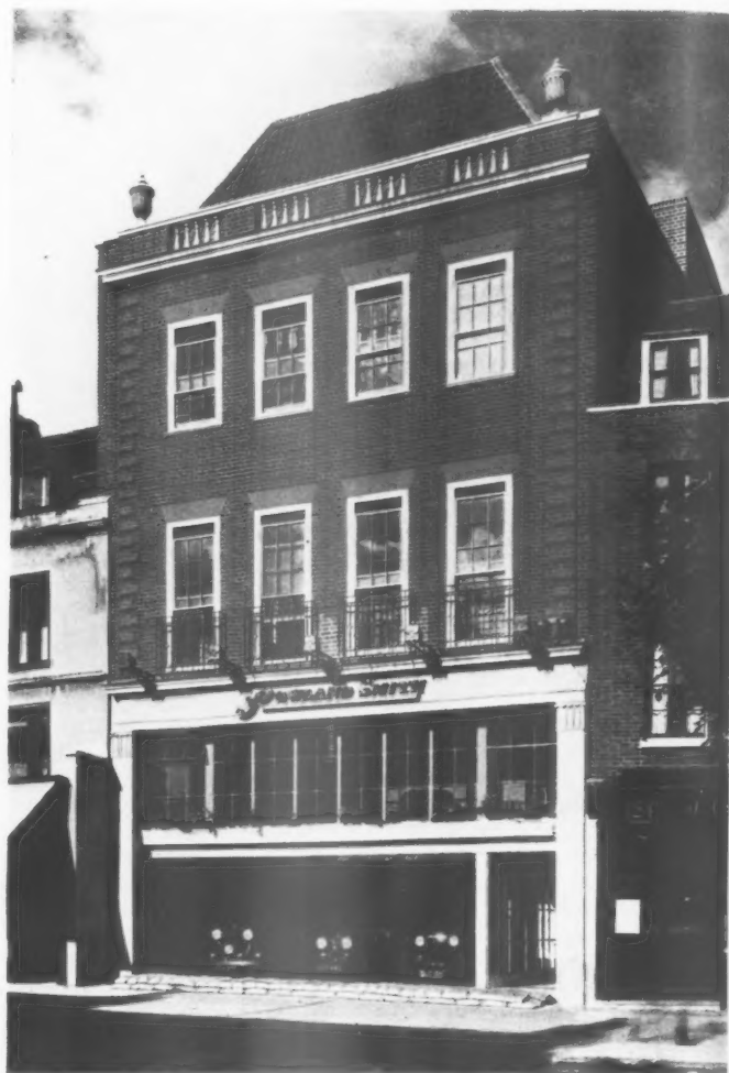
The main front. The flood-light brackets at first floor level are of wrought-iron.
