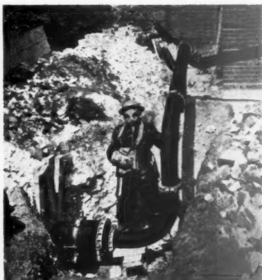
System of temporary connections for fractured mains described in question 187.
