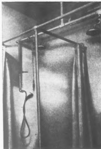
Plant for providing hot water showers for a decontamination squad consisting of 18 men. From “A.R.P.: A Job for the Gas Industry.”
