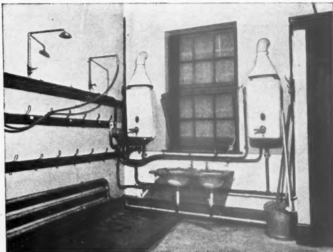
Instantaneous gas water heaters in a public Cleansing Depot. From "A.R.P.: A Job for the Gas Industry."
