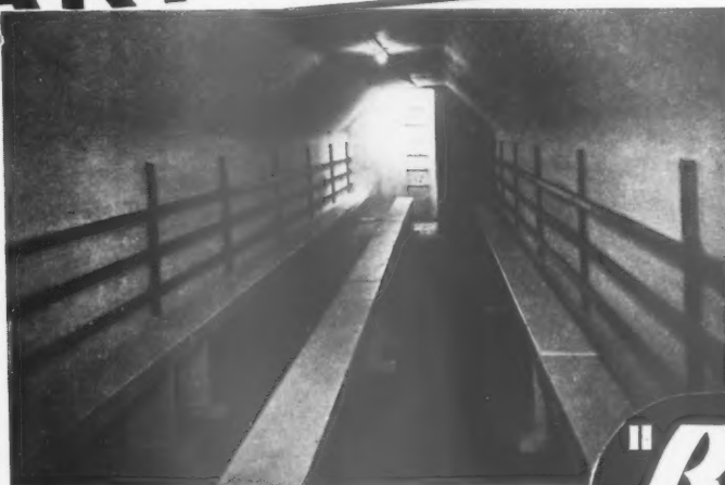
Interior view of a typical Air Raid Shelter constructed with Concrete and "Ribmet" Reinforcing Units.
