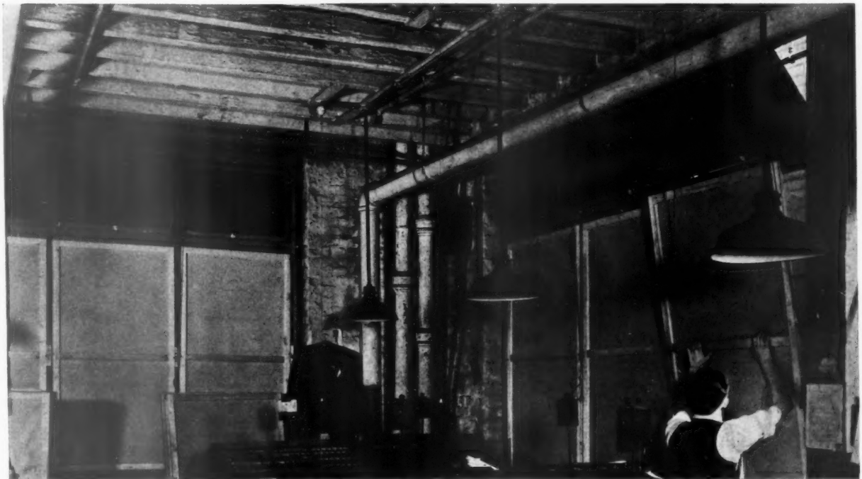
Blacking-out in a London workshop. In order to make the blackout effective the fanlights used for daytime ventilation must be closed, and only the use of screened extract fans prevents steady deterioration of the atmosphere.
