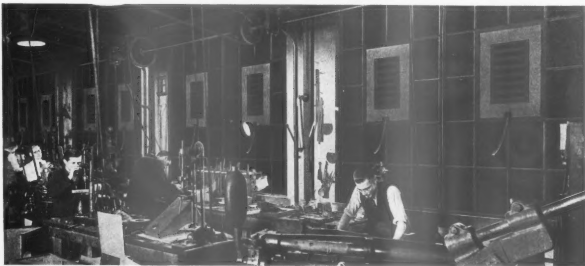
Louvred blackout ventilating panels inserted in workshop windows.
