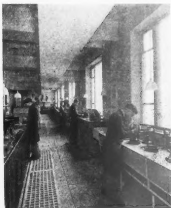
Top, the pathology and research laboratory on the second floor in the west wing. The window, which is standard throughout the building, consists of a large plate-glass centre in a wood frame with metal hoppers and casements at the sides. Above, left, mechanical laboratory; right, a recovery room adjoining the extraction room.
