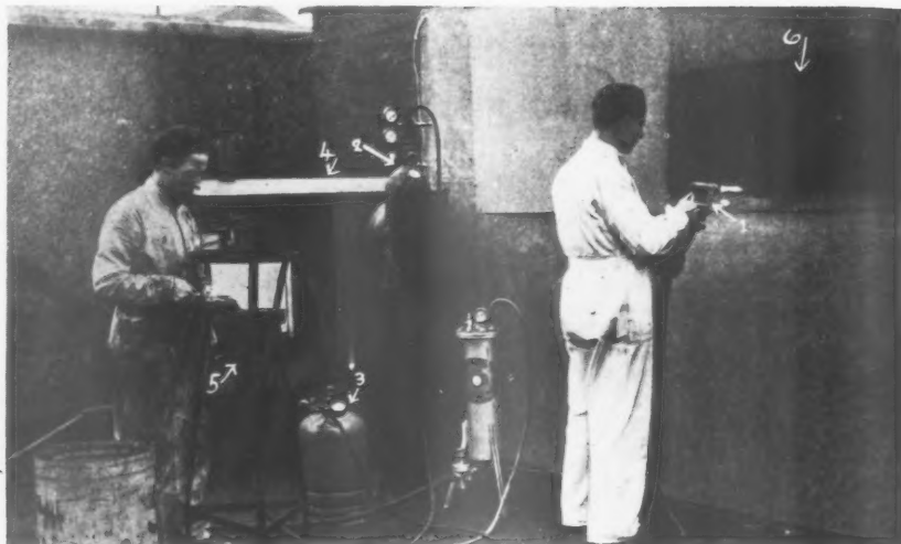
The application of "gunned" asphalt:—1. The Flame-gun in the hands of the operator. 2 & 3. The Compressed Oxygen and Propane Supplies for feeding the flame to the gun. 4. A normal type of portable compressor for supplying compressed air to the gun, by means of which the powder is sucked through a supply pipe-line in partial vacuum from the feed hopper (5). 6. Shows the asphalt coating already applied in a continuous layer.
