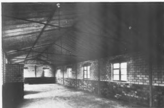
New Army hut, showing the Bison (pre-cast concrete) roof in position.
