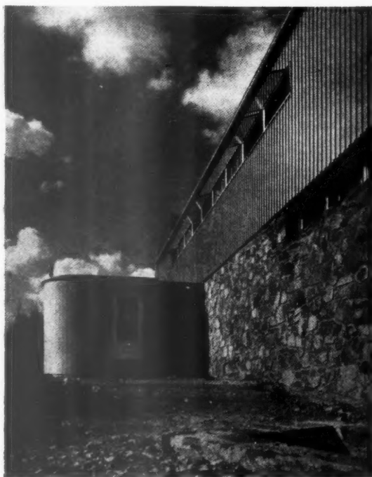
The above photographs show the entrance unit in built-up flush boards and the cantilevered stair to the roof deck
