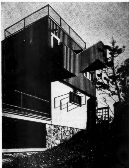
The above photographs show the entrance unit in built-up flush boards and the cantilevered stair to the roof deck
