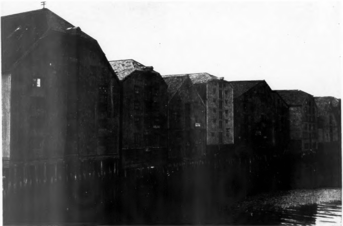
The timber granaries lining the harbour at Trondheim, Norway, are built entirely on wood piles and are painted in various shades of orange, red and yellow.
