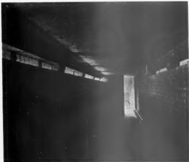
Glass bricks in A.R.P. Left, giving natural light to a surface shelter and, right, to a warden's post
