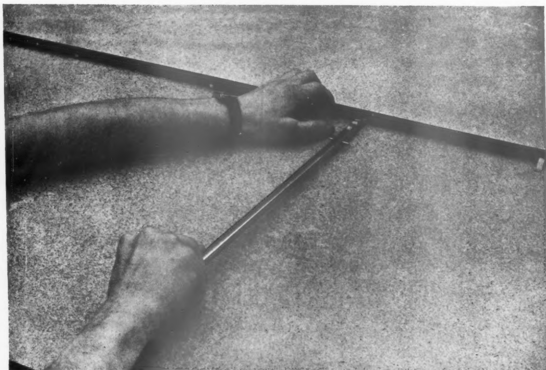
Inserting the spring clips in the slotted metal cover strips.
