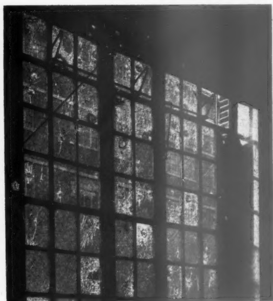
Left, wired glazed window pierced by bomb splinters. The velocity of the splinters and the relatively little damage done by them and the accompanying blast to the glass may be judged by the holes made by the splinters in the cast iron framing and infilling panel above.
