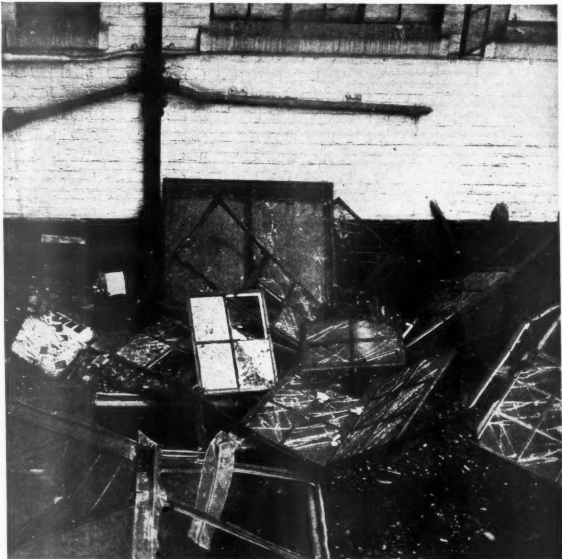
Steel casements in an area after having been pulled from a fourth floor window by the suction wave of a near miss. Most of the wired glass has remained in the frames after the explosion and a forty-foot fall.
