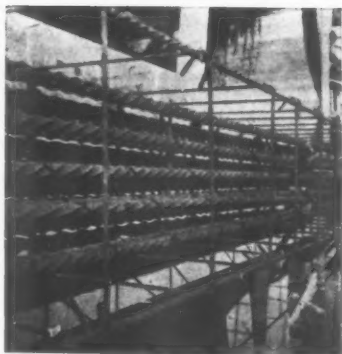
Square Grip Heavy Section Bars in position
