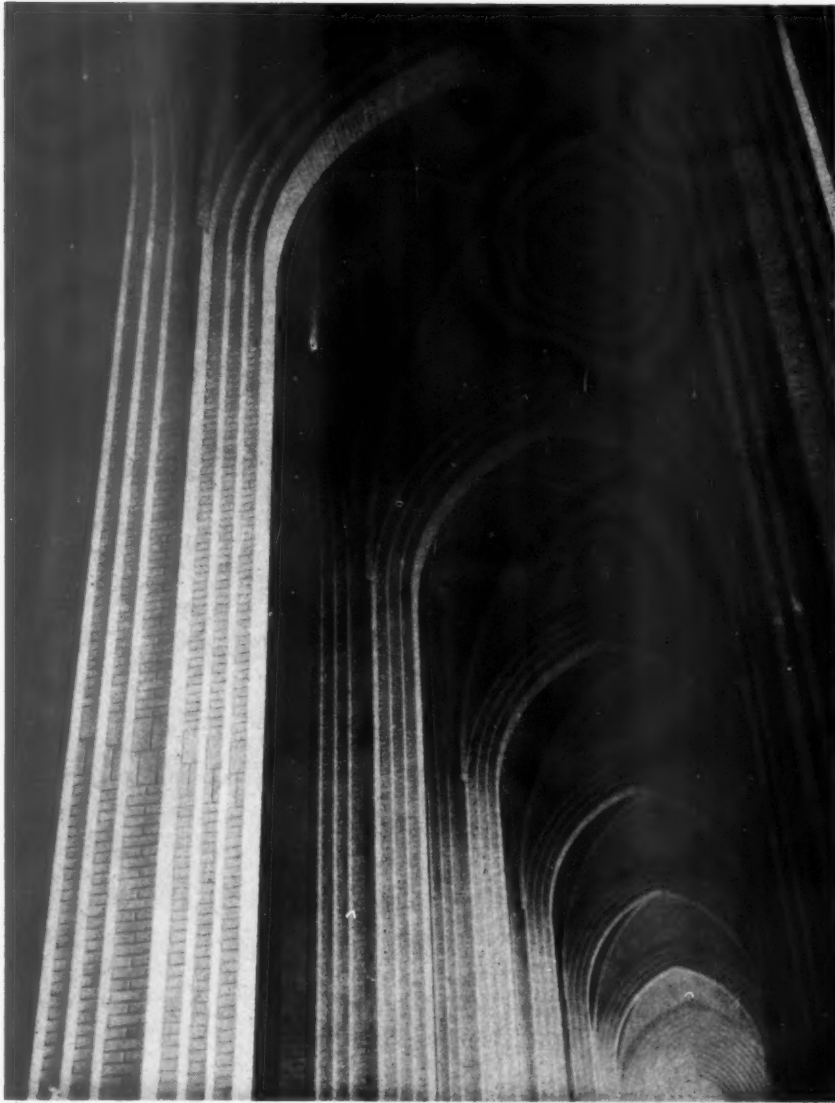
Brick vaulting in a memorial church at Copenhagen. The whole of the structure, internally and externally, is carried out in a light coloured common brick.
