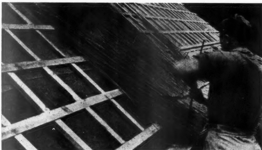
2: Wedging the first layer of reed tight under the hazel, which is then secured with an iron spike to the batten.
