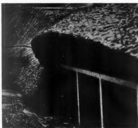
4: The sweep round the dormers and the second layer of reed in position.
