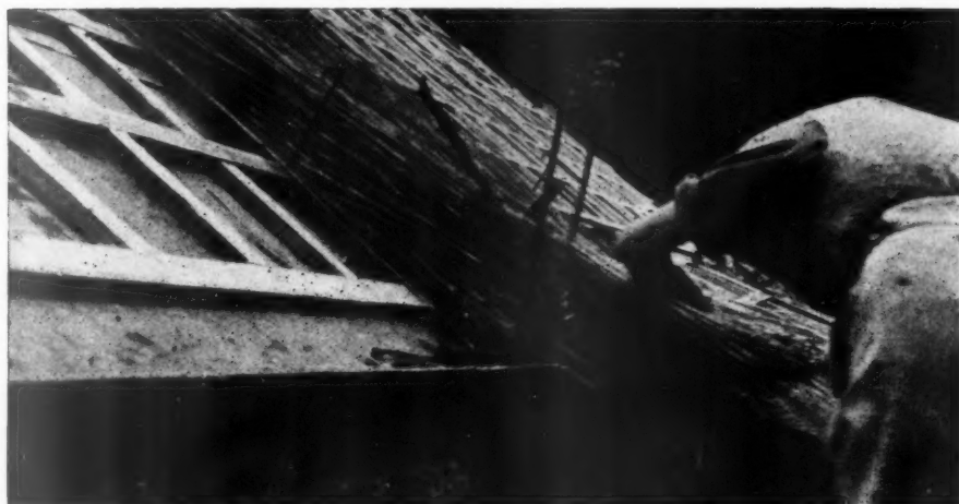
1: The tilting fillet at eaves level and the first layer of Norfolk reed thatch being placed in position.
