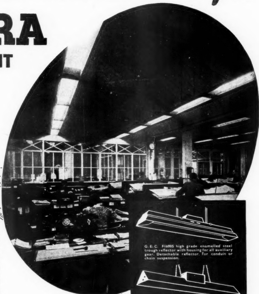
G.E.C. F16907 enamelled steel trough reflector with housing for all auxiliary gear. For conduit or chain suspension.
