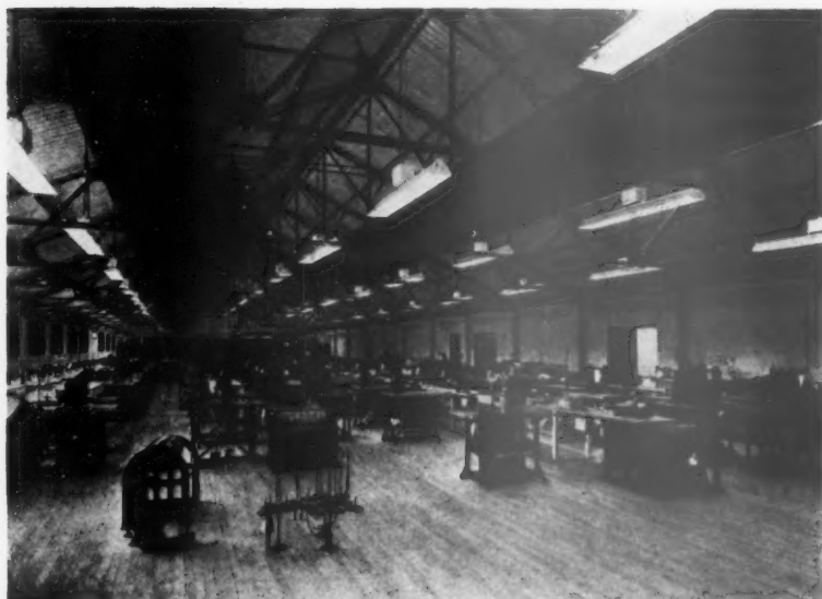
A fluorescent factory lighting installation by Edison Swan Electric Co.
