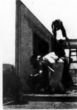
4 One wall already up, workmen tighten connections.
