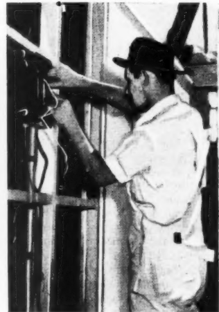
7 Electrician puts in wiring without waiting for roof.
