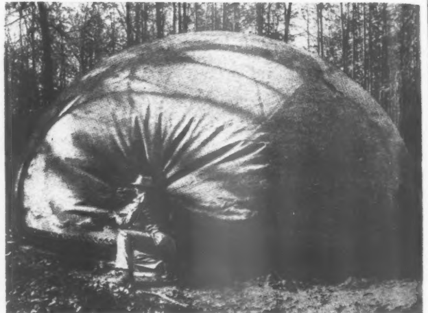
2 The balloon is made fast to the circular foundation with ropes and iron bars. Air is pumped into the balloon at 1 1/2 lb. pressure by the same compressor later used to apply the concrete. The inflation time is 5 minutes.
