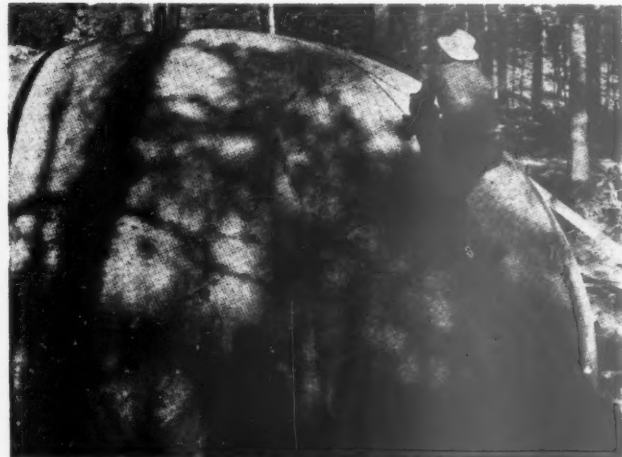
3 A 900 dollar canvas balloon with rubber coating inside and out is used as "pneumatic form." Door and window frames are placed flat against the balloon and sealed into place as the concrete goes on.
