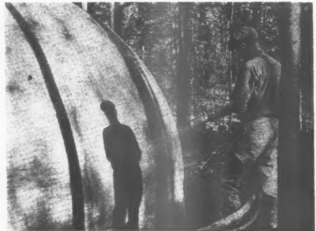
4 The first cover of concrete is 1 in. thick and becomes the inner wall of the house. Then comes layer of insulation (asbestos and cellulose) followed by 2 in. outer wall of concrete. The process takes 7 1/2 hours.
