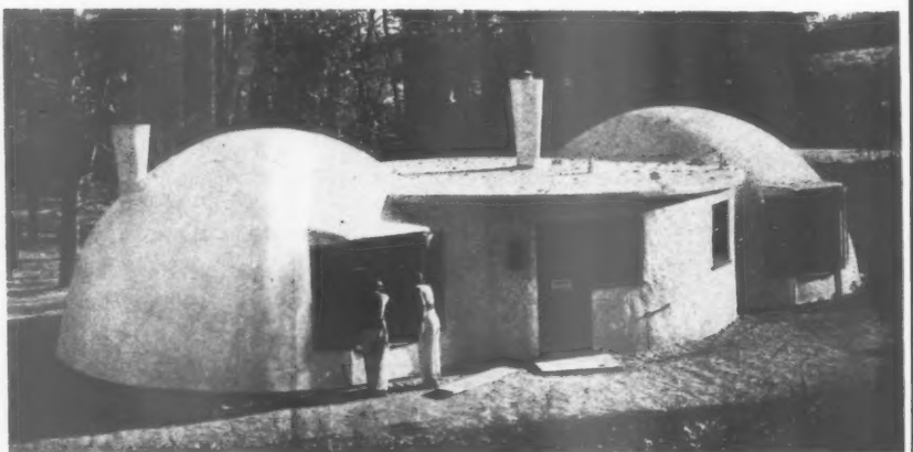
A double balloon house with connecting foyer, containing a living room 14 ft. by 23 ft., brick fireplace and bookcases, two bedrooms each 14 ft. by 10 ft., kitchen 9 ft. by 10 ft., bathroom 8 ft. by 8 ft., and nine closets. The house uses gas for heating and the bath is fitted with a shower.
