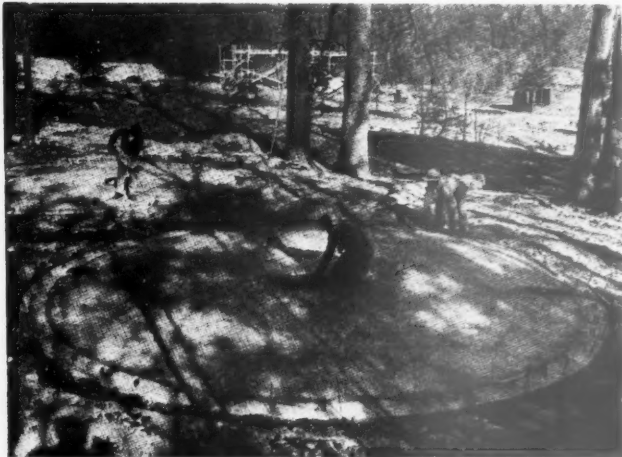
1 The ring-shaped foundation of the balloon house is 6 in. below the frost line. An 8 in. concrete floor is laid over an 8 in. gravel base. Wood flooring is laid last, after the wiring and pipes are installed.
