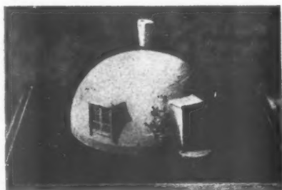
Model of a one-dome "bubble house," made from a balloon and referred to in Astragal. Such houses could be made quickly and in large numbers to shelter war-evacuated populations of American cities. Other illustrations of balloon houses and notes on their construction are on page 74. All the pictures are reproduced from Life .
