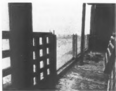
The Penilee Housing Scheme is illustrated in this issue. Above is a detail of balcony access gallery in a tenement block. Note pre-cast concrete panel units.
