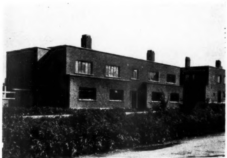
Above—general view of two-storey cottage block. The chimneys do not smoke. This is due to the special precast concrete chimney cappings and also to the fact that the top of the chimney is always designed to be 15 ft. above the springing of the arch of the topmost fireplace opening, i.e. 7 ft. 6 in. above the flat roof. Left—detail of entrance to two-storey cottage type house. Note the concrete copings and window sills. The door canopies throughout the scheme are of concrete.
