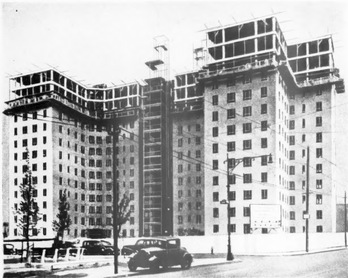
This brick-faced, reinforced concrete building at Brooklyn Navy Yard contains housing accommodation for 207 families. It was completed in a little over five months.
