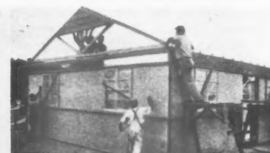
12. An end roof truss, equipped with ventilating louvres, is fitted into position.
