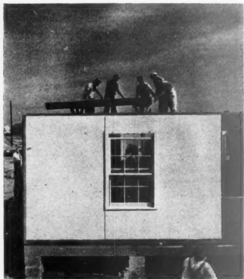
5 8.25 a.m. Removing a ceiling panel. All ceiling sections were removed by 9 a.m.
