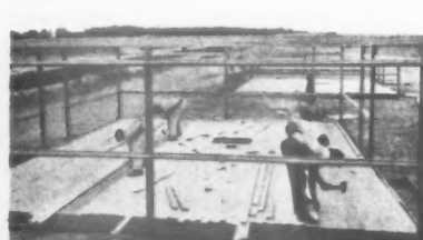
8. The floors are laid with 1 1/2 in. thick T and G flooring.
