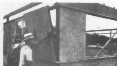
10. A short Cementos board panel is put into place at the corner of window course. Board is nailed to wood columns.
