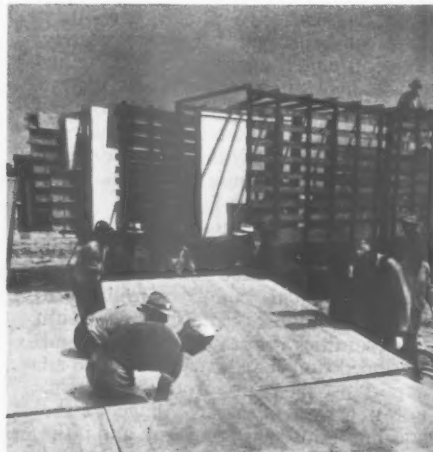
8 9.45 a.m. Last wall section was down and on the truck by 9.40 a.m. Here the floor panels are being removed.
