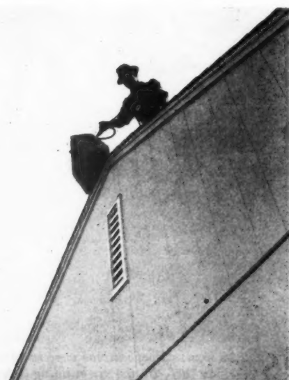
14 12.35 p.m. The mason about to start work on the chimney. Here he is seen hauling up chimney block.
