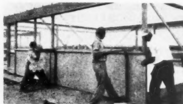
9. A sheet of 1 1/2 in. Celotex Cementos board is being applied to the lower section of a wall. Panel is 12 ft. long x 4 ft. wide.
