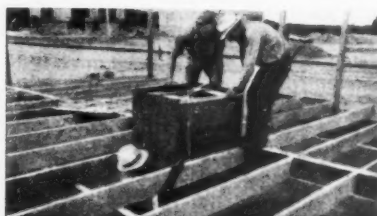
7. An oil-burning furnace is put into each house before the flooring is laid.
