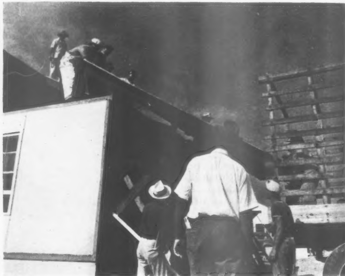
6 8.35 a.m. Roof pieces being lifted off the house directly into a truck which had been brought to the side of the house.
