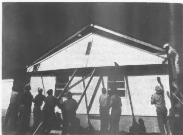
4 8.10 a.m. One of the gable ends is being removed; gable ends were dismantled in approximately twenty minutes.
