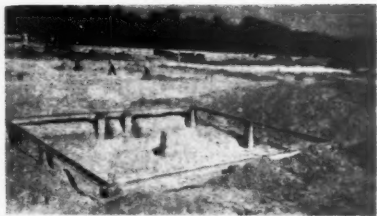
1. Each house rests upon concrete piers and precast concrete rails.
