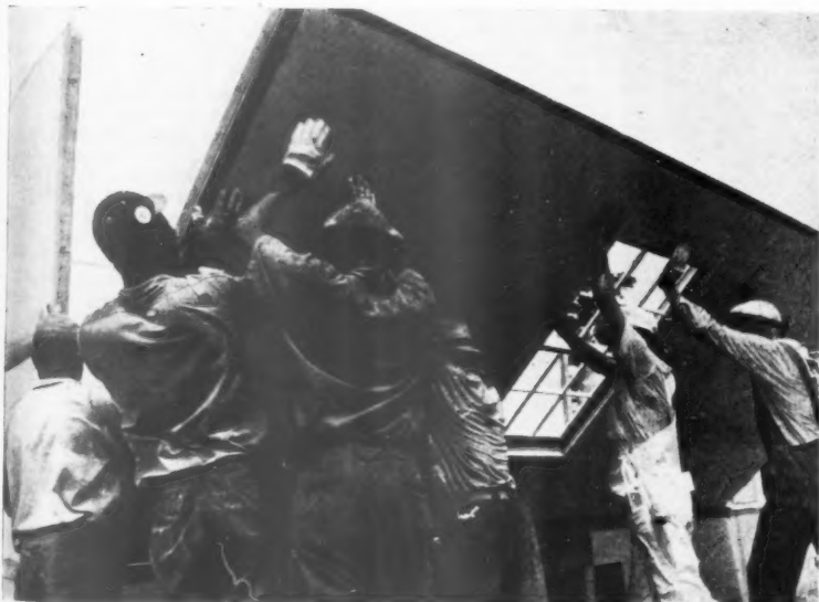
13 12.15 p.m. One of the exterior wall panels being lifted into position. In this illustration it will be seen that the window frame was left in position when house was dismantled.
