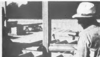
4. The window course sills fit into recesses in the wood columns. The sills are also a millwork product.
