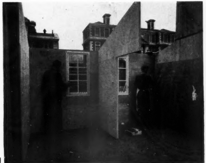
10 Section showing CONSTRUCTION. Note absence of roof trusses and beams.
