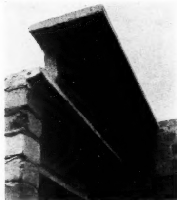
Detail of typical precast stair unit ; right, standard units in position in staircase. Below, typical entrance to block of flatted houses.
