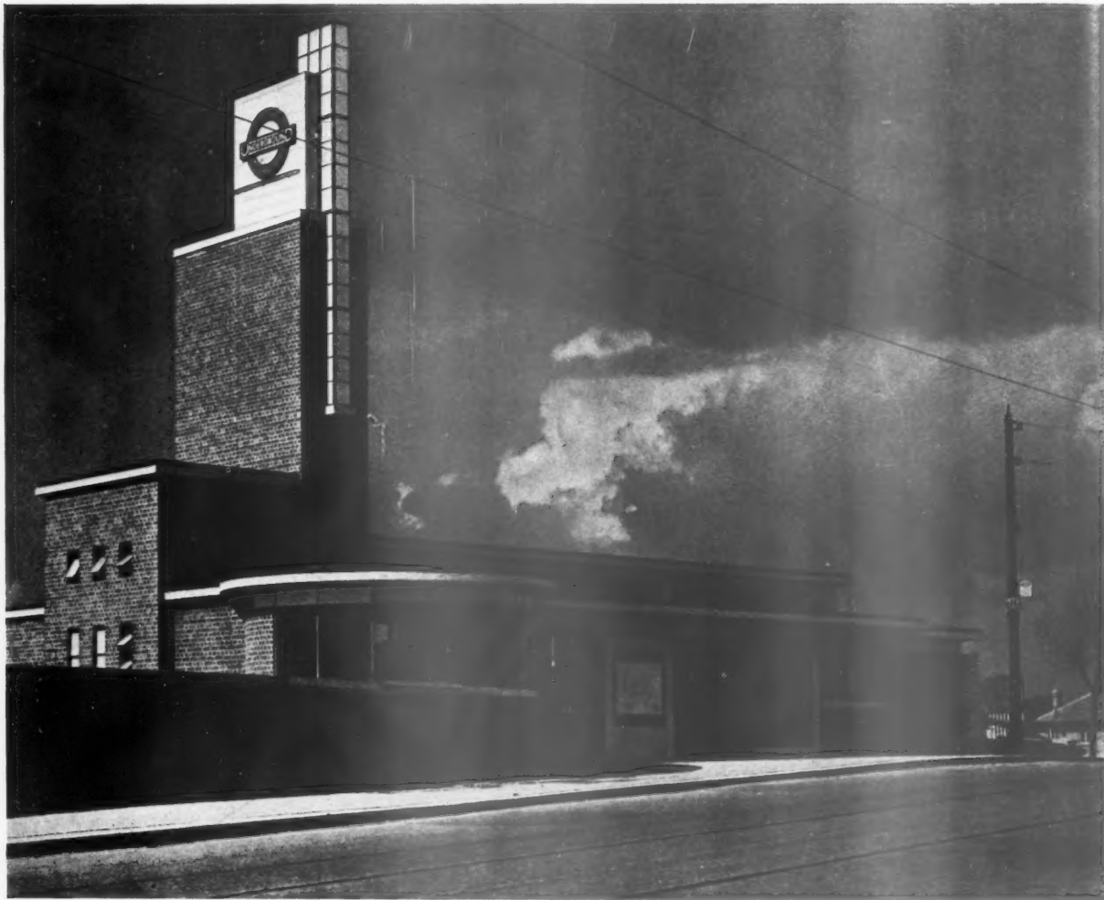
Above and below, Boston Manor Station, designed by Adams, Holden and Pearson. Built in 1932, this is one of the smaller stations along the western extension of the Piccadilly District line. Building is carried on steel girders over the track. Tower is carried up in brickwork, 18 ft. 6 in. above the roof of the booking hall and is finished with a tiled blocking carrying the bull's-eye sign, with a glazed lighting column for publicity. Right, louvred self-closing sheet steel doors to lavatories at South Harrow Station.
