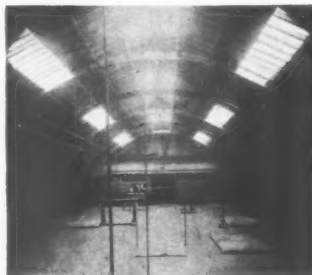
The gymnasium built for the Gordon Institute for Boys in Liverpool about 1890. The building, which measured 110 ft. by 56 ft., was to cost only £1,000. The area is spanned by ten semi-circular wooden arches rising on either side directly from the ground. They carry the roof as well as the gymnastic apparatus, an ingenious arrangement, as the curves of the arches distribute all strains, and the elimination of all angular joints makes the construction ideally safe.
