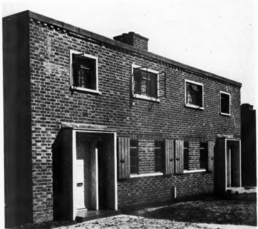
Semi-detached blocks. The A.R.P. shutters are, of course, removable after the war. Facing page: top, perspective view; the Staff Houses are on the right. Bottom, view showing the use of the long terraces; the end units in each terrace are pairs of flats.
