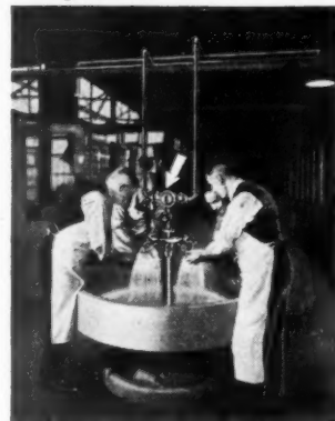
Leonard-Thermostatic hot and cold Water Mixing Valve supplying ablution shower for workers.
