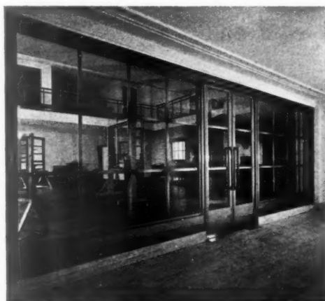
This surround is constructed of pressed metal framing. The panels are filled with glass.
