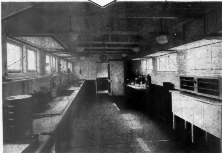
Laboratory of wood-framed construction with Gypklith rendered on the exterior, and Gyproc for the interior linings.
