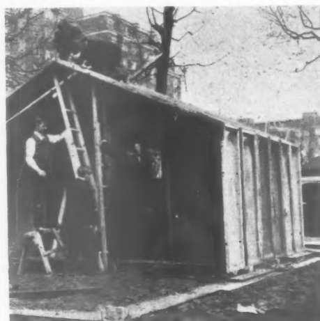
Patrick Portable Building. —Temporary hutments are required for many war-time purposes, and the problems of their construction have produced many ingenious systems. In this example, the sheet filling is formed in the framework, and its strength plays an essential part in the structural system. The units are 24 in. wide, and span from the foundation to the ridge in one length. The section of each unit is formed in the shape of a U, and its greatest depth is at the eaves. The units are made of concrete and are reinforced by sackings. This system was designed by Mr. J. H. de W. Waller.
