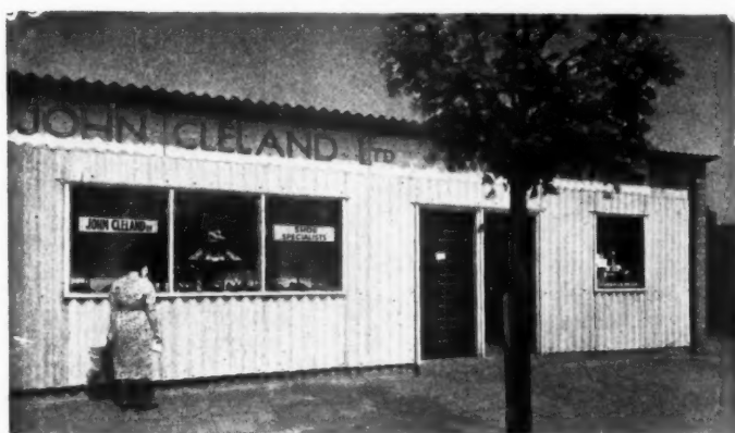
Temporary Shops at Coventry. —The bombing of important cities and towns has caused widespread destruction in many essential shopping areas. The City Architect of Coventry has built about forty temporary shops in the centre of the town to provide accommodation that will fulfil minimum requirements until such time as the new plans for reconstruction have been brought into effect. The shops are constructed of a light framework and are surfaced on all exposed areas with impervious sheet asbestos-cement materials. Roof and wall covering sheets are corrugated to simplify the framing requirements, but flat sheets have been used over the fascia areas to provide an untextured base for the shop signs.
