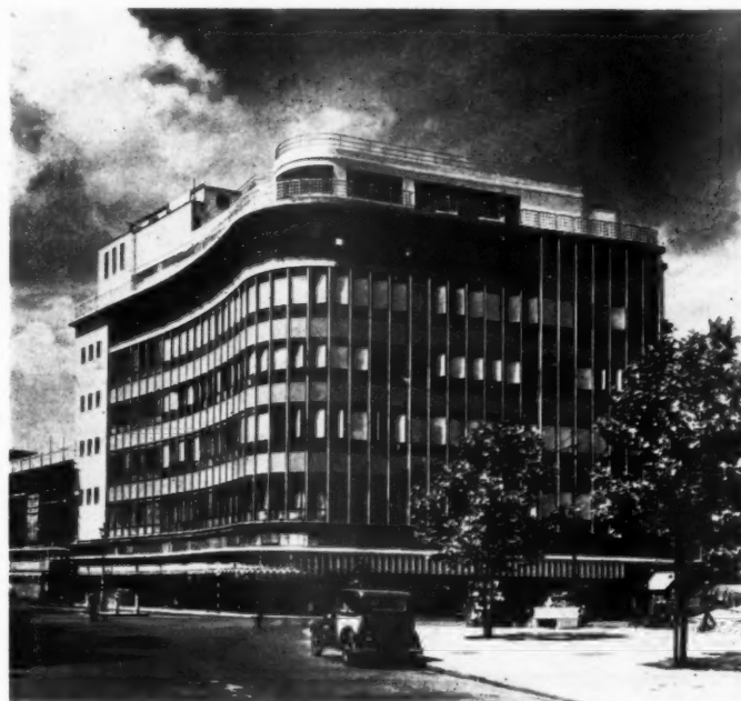
Peter Jones' Store, Sloane Square, S.W. —Before the war, sheet materials were used extensively on the street frontages of large store and office buildings. In this example, glass sheets have been fixed over the whole area of the external walls, and colour variations are obtained by changing the backing sheets suspended in the cavity behind the glass. Facing page: Interior of asbestos-cement curved hut.
