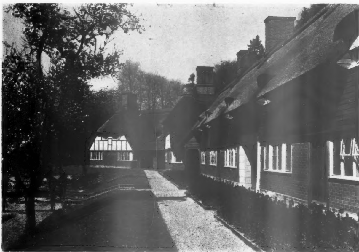
Two views of the south front. On this front the roofs are covered with Norfolk reed thatch; they are tiled on the north side. Facing page: close-up of the centre of south front.
