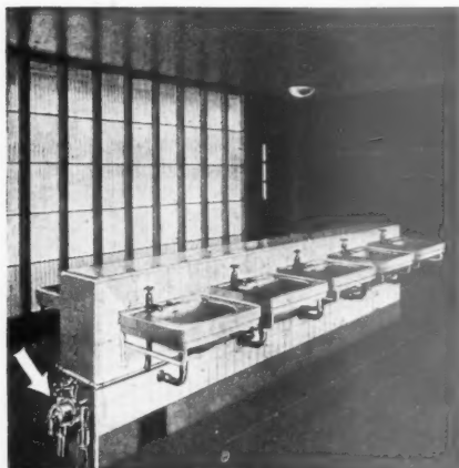
Leonard-Thermostatic hot and cold Water Mixing Valve serving a range of washbasins.
