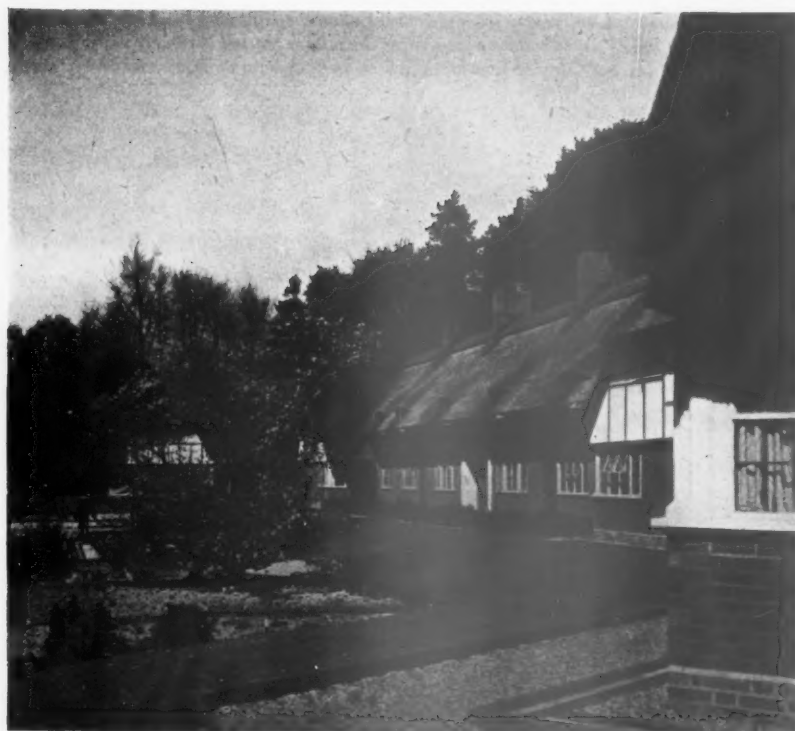
Two views of the south front. On this front the roofs are covered with Norfolk reed thatch; they are tiled on the north side. Facing page: close-up of the centre of south front.
