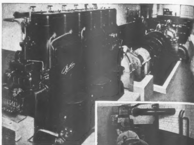
Photographs show Petter Engines in- stalled for electric gen- eration and pumping.
