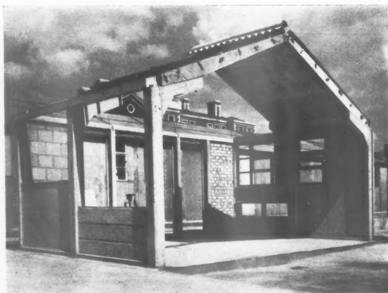
Photograph showing the MOWP, type 1, hut during course of construction.
