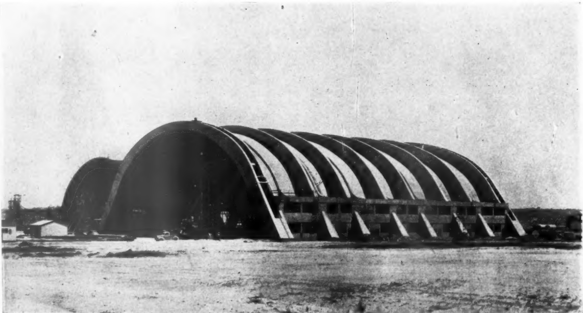
This reinforced concrete hangar, 294 ft. span and 81 ft. high, is being built at San Diego, U.S.A.
