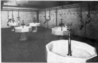
Leonard-Thermostatic Hot and Cold Water Mixing Valves serving ablution fountains.
