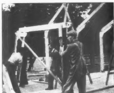
5 The small crutch is held in position and a small "A" frame is ready for the next lift.
