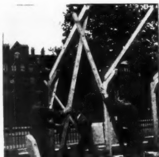
8 Large "A" frame is inserted. The ridge pivot is lifted as high as possible.
