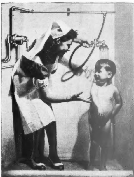
Leonard-Thermostatic hot and cold Water Mixing Valve serving a shower at a day nursery.
