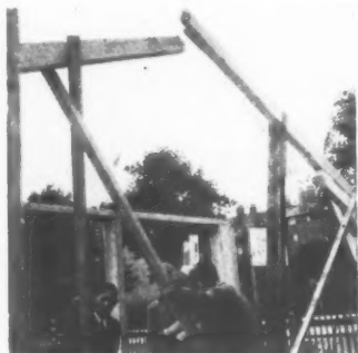
6 The remaining half-frame is erected similarly to the first half frame. Wedges are inserted.
