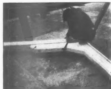
2 The stanchion and rafter are laid horizontal and the bolts fitted by one of the workmen.
