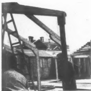
4 The frame is lifted and the "A" frame is inserted under the bracket of the stanchion.
