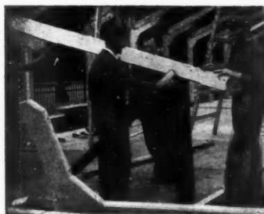
7 Frame is lifted and temporarily supported by a piece of timber and a small crutch is ready for next lift.
