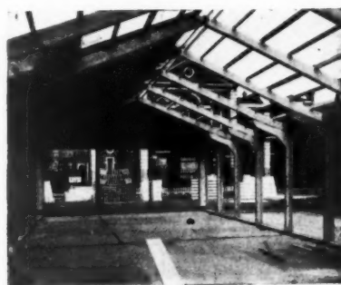
11 Partially completed roof, showing wiring on of purlins.
