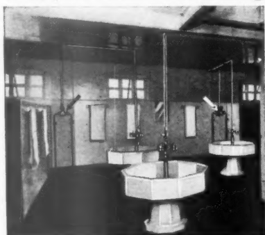
Leonard-Thermostatic hot and cold Water Mixing Valve serving ablution fountain.
