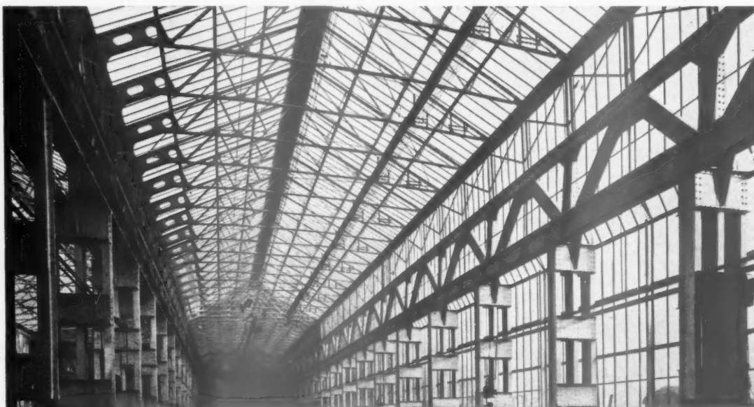
Bay of a machine shop glazed with \frac{1}{4} " Rough Cast Double Rolled.
