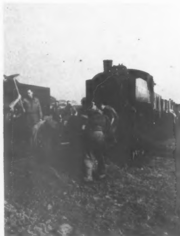
Left, Sappers laying the last part of the railway track; it is 25 miles in length and took 3 months to complete. Right, Trench excavator. This digs a 3 ft. 6 in. trench for water-mains at a speed of half-a-mile an hour.
