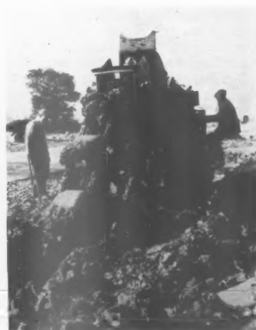
Left, Sappers laying the last part of the railway track; it is 25 miles in length and took 3 months to complete. Right, Trench excavator. This digs a 3 ft. 6 in. trench for water-mains at a speed of half-a-mile an hour.
