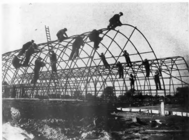
Erecting an Iris hut for storage and workshop. It is of tubular steel construction.
