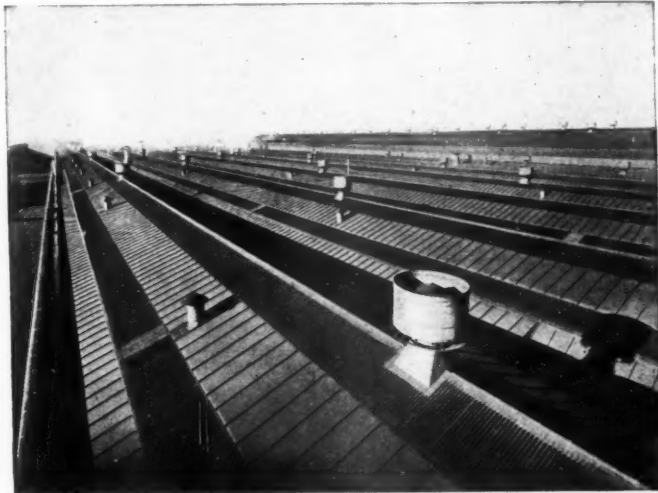
A typical installation showing the extensive use of Wired Glass in a factory roof.
