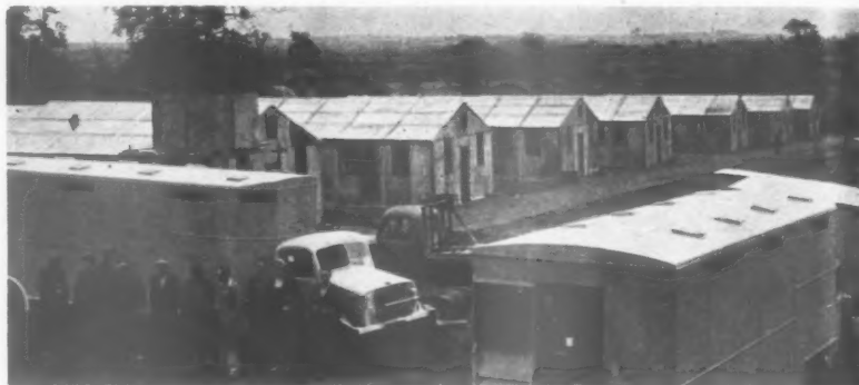
The prefabricated huts (3 dormitories, 1 canteen, 1 store and 2 offices), built by MOWP's mobile builders to house the advance party of workmen of the main contractor.
