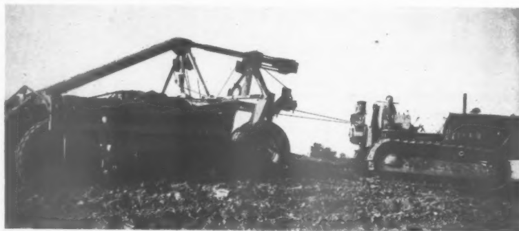
Twelve cubic yard scraper for road making. It does the work of 400 men—400 ft. by 12 in. deep in 90 minutes.
