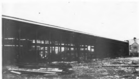
Exterior of the outside wall of the same classroom; and the general classroom wings at a later stage, with glazing bars and weather-boarding. It will be seen from these two photographs that the structure is not concealed, but constitute the design.
