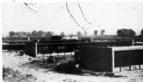
Exterior of the outside wall of the same classroom; and the general classroom wings at a later stage, with glazing bars and weather-boarding. It will be seen from these two photographs that the structure is not concealed, but constitute the design.
