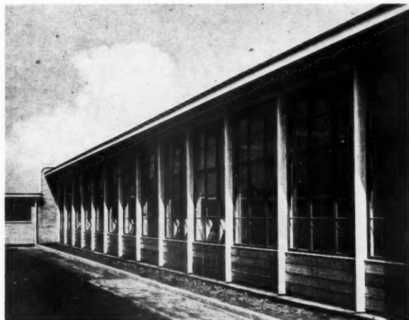
Not only is the exterior pleasant, but the light steel framework, filled with glazing, gives a light appearance to the whole structure.
