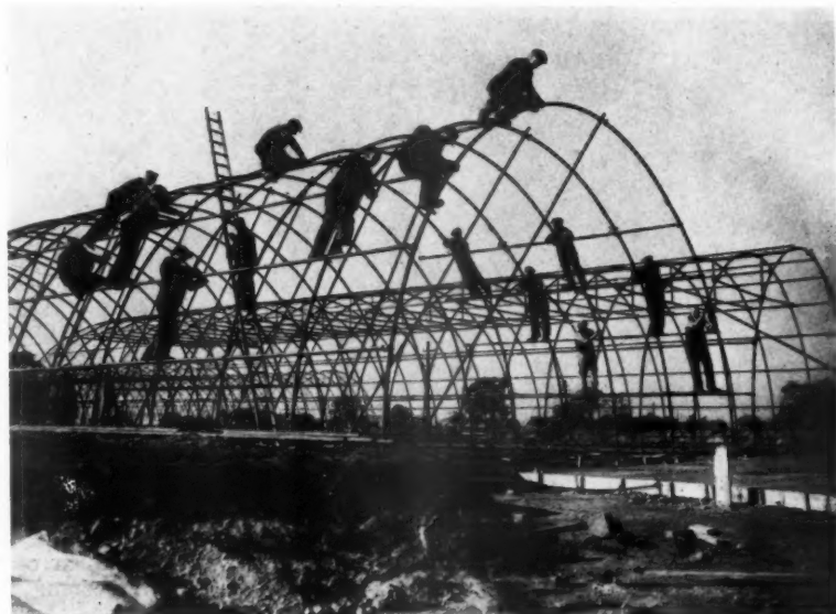
War Office Camps for the American Army in this country were approaching completion this month. Records in speed of erection were broken by full use of mechanical road makers, trench excavators, a battery of concrete mixers and efficient organization. The Iris tubular steel form of construction was used for storage huts and workshops.
