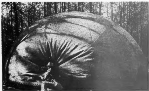
A Village of Bubble Houses, designed by architect Wallace Neff, built near Washington and financed by U.S. Government. General structure is concrete sprayed onto inflated balloon of rubber-coated canvas.
