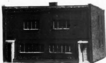
Coventry Shelter-to-House Scheme. A scheme to build air-raid shelters convertible in peace time to small houses was officially approved in principle. The structure of the shelter is practically unaltered when it later becomes the ground floor of the future house.
