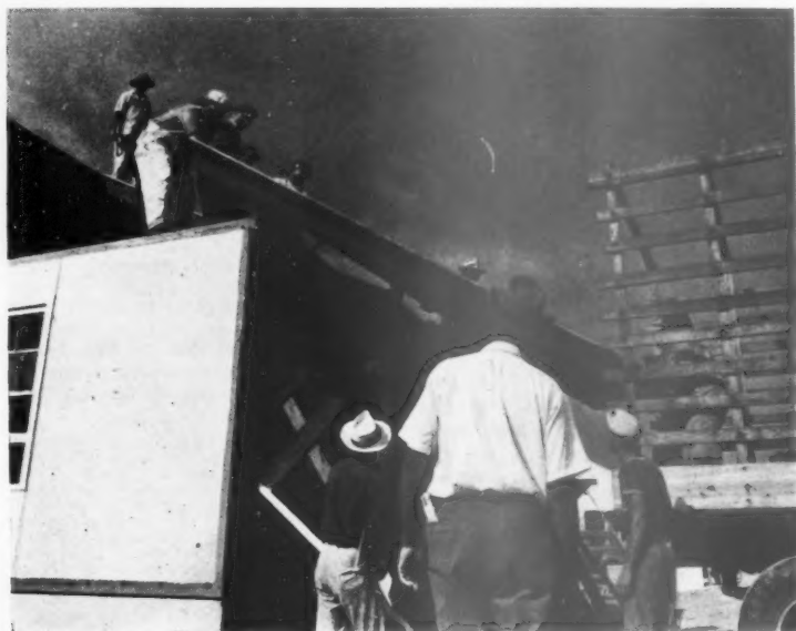
Mobility and Pre-fabrication in Housing, stimulated by war needs, have formed the greatest technical developments of the year, especially in the U.S.A. Here is a demountable house built at the U.S. Navy Powder Factory at Indianhead, Maryland. Demounting, transport of 40 miles and re-erection of hut took less than seven hours.
