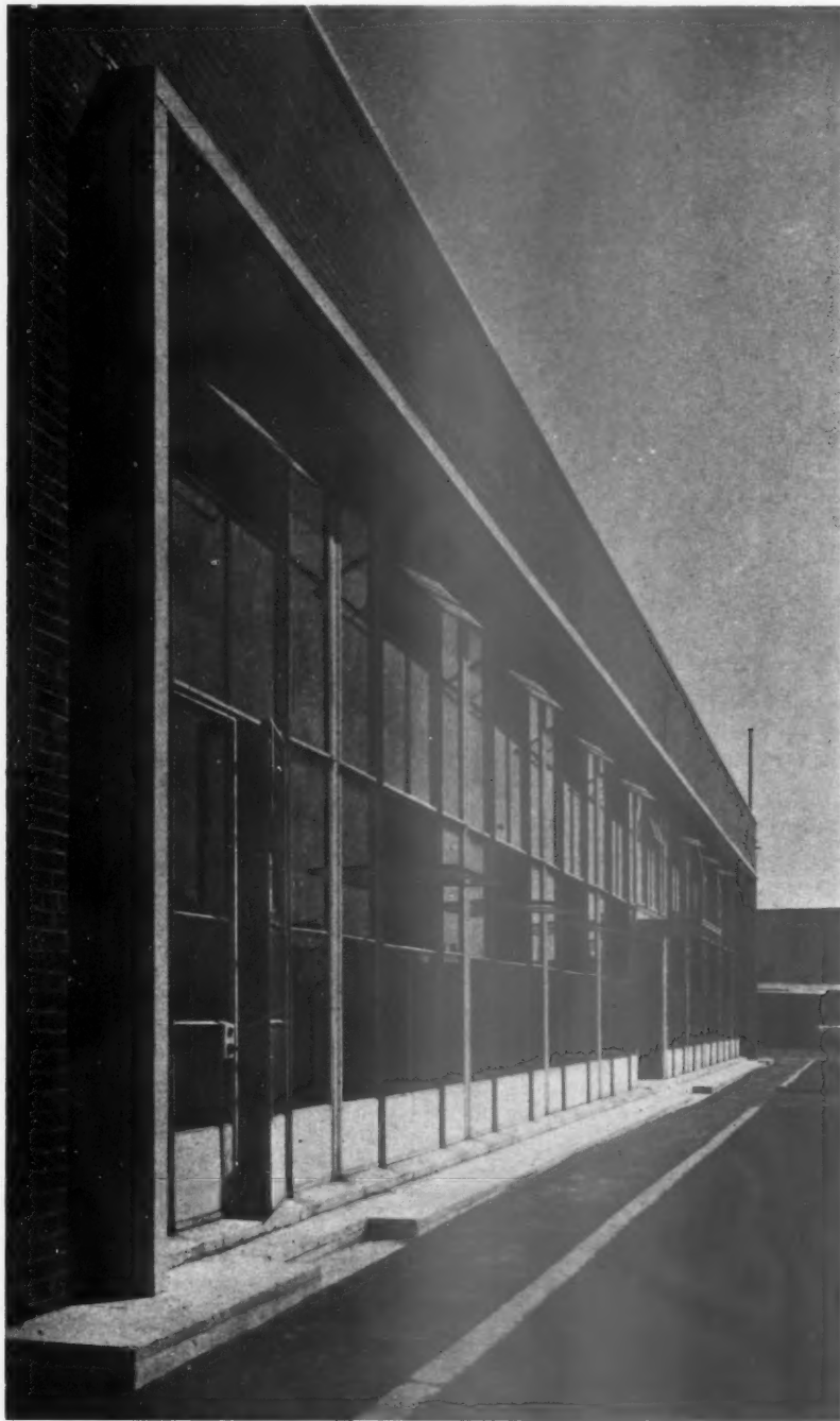
Above: The assembly halls are steel framed with 11 in. cavity walls, faced with buff-coloured cement bricks. Right: a general view of the school from the north-east.
