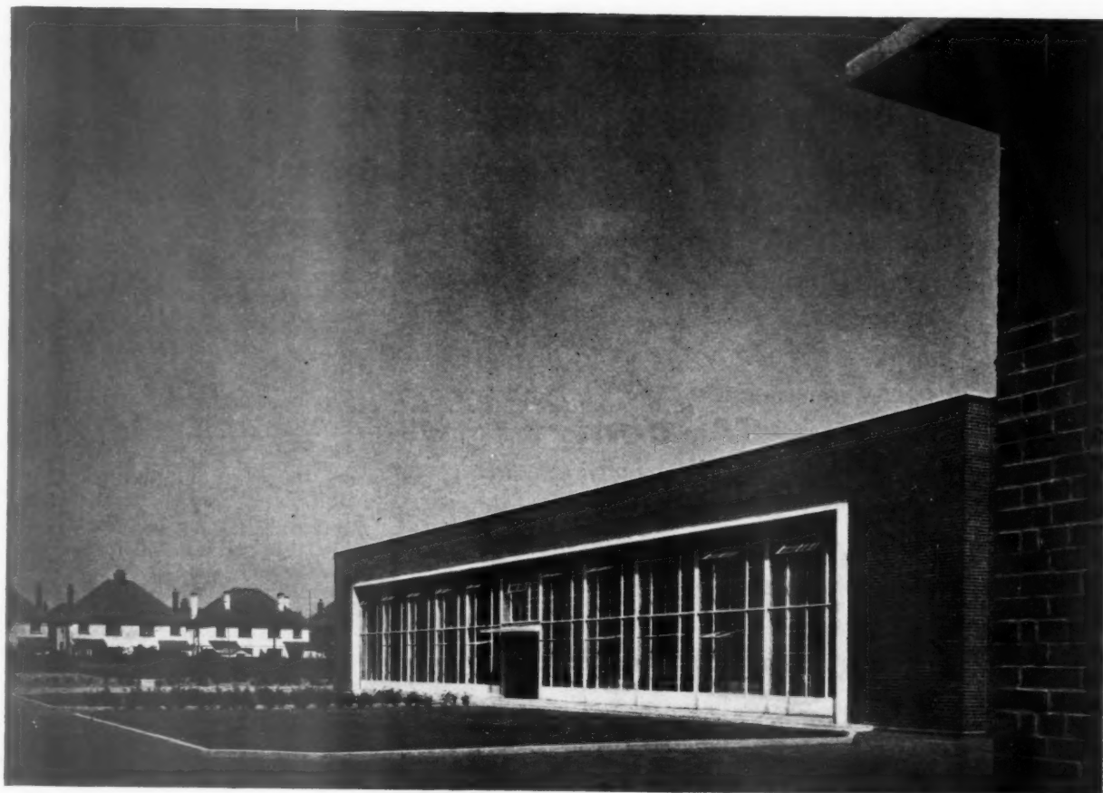
View of the assembly halls looking north-east.
