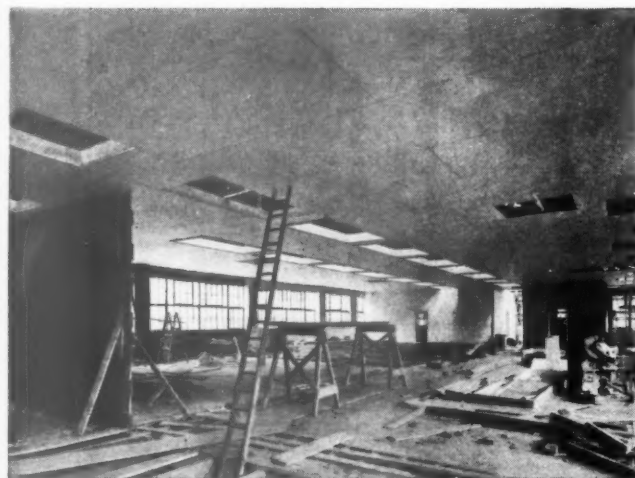
Gyproc ceilings being erected at Woolwich.
