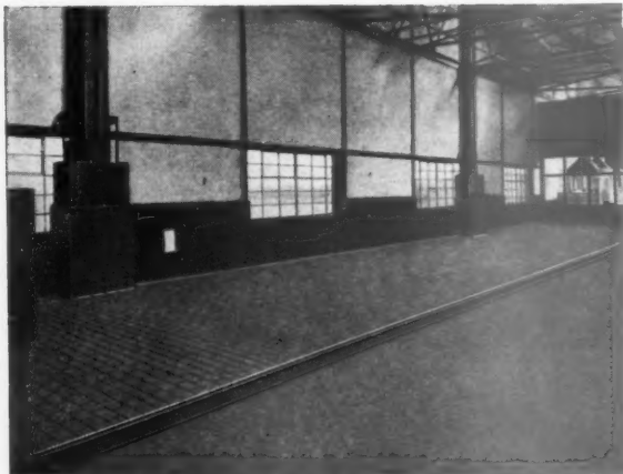
An Acid-proof Floor laid by Prodorite Ltd.
