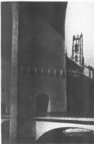
Two bridges with an uncovered concrete finish. Left, the Pont de Pérolles at Fribourg, Switzerland, having a bush-hammered finish. Centre and right, the Traneberg Bridge, Stockholm, with a finish formed by timber boarding.
