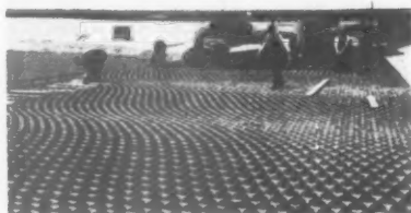
Creosoted timber base of a Delaware Bridge. Triangular plates, called Shear Developers, are embedded in the concrete slab.
