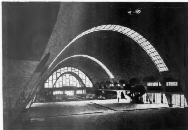
Rheims Market Hall, designed by Maigrot; an example of thin-shelled concrete vaults (From Pencil Points , January, 1943). See Information Centre, Item 1159, on this page.
