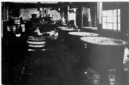
A Prodorite Acid-Proof Floor laid at a large Food Factory.
