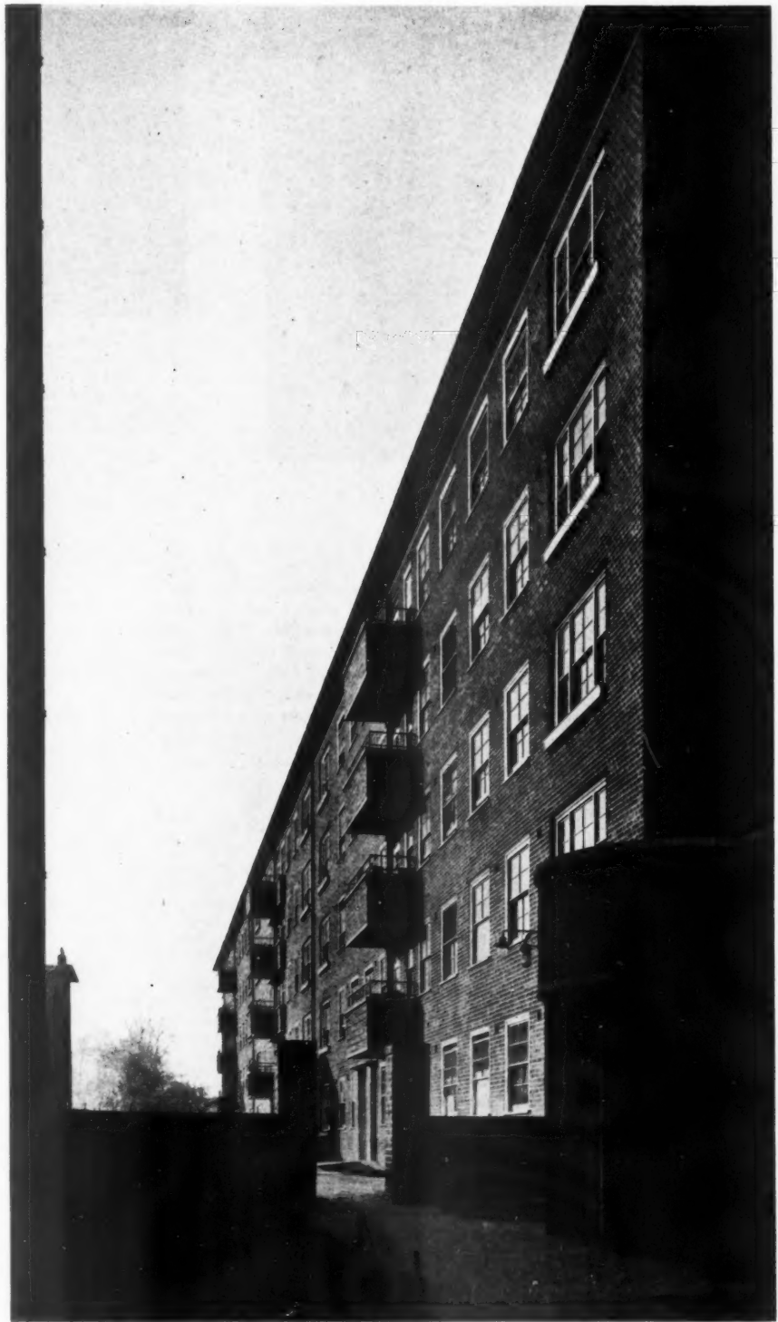
A view in a quadrangle at Springfield. External walls are 14 in. thick, faced with sand-faced multi-coloured bricks in dutch bond.
