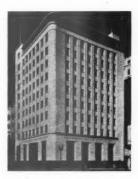
Top, in the banking hall the ledger clerks' and tellers' cubicles have low glass screens without grilles. Above, general view of exterior which is faced in Stawell freestone; the main entrance is in the Collins Street front, which is shown on the left of the illustration; the other elevation faces Elizabeth Street. Below, plans of ground, second, third and ninth floors.
