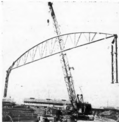
Left (top), timber bents 79 ft. wide and 52 ft. high, designed as fixed end rigid frames: columns were laced together in pairs to provide lateral rigidity against buckling. Above, bents of 100 ft. span bowstrung trusses and 25 ft. columns erected with a crawler-crane. Left, two-span bents, 200 ft. long, 35 ft. high, erected by three crawler-crane operating simultaneously. See item No. 1244.
