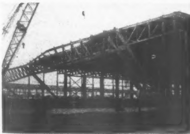
Left (top), timber bents 79 ft. wide and 52 ft. high, designed as fixed end rigid frames: columns were laced together in pairs to provide lateral rigidity against buckling. Above, bents of 100 ft. span bowstrung trusses and 25 ft. columns erected with a crawler-crane. Left, two-span bents, 200 ft. long, 35 ft. high, erected by three crawler-crane operating simultaneously. See item No. 1244.
