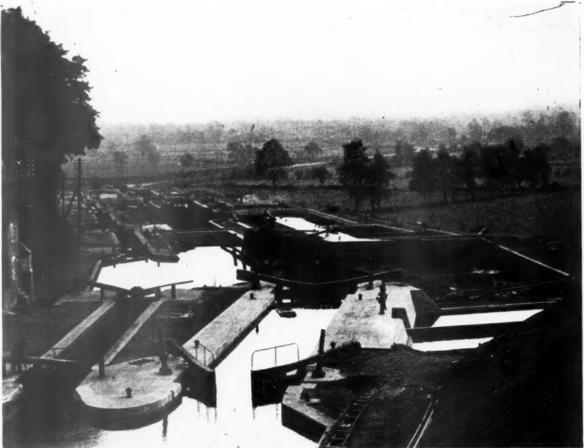
Reconstruction of canal lock in reinforced concrete.
