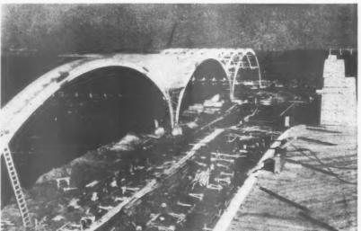
Some of the longest laminated timber arches ever erected at a USA airbase, Arches are of 7½ ins. by 39½ ins. cross section. See No. 1393.
