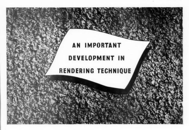
EXTERNAL renderings finished with a rough texture do not crack or craze or show blemishes like smooth surfaces.
