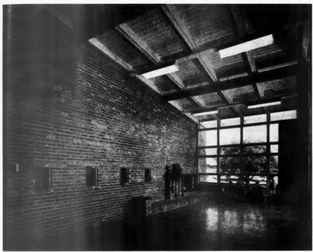
used from a previous school, demolished in the district, were incorporated in the new one. The brick is new; it is reddish brown in colour, and is left unsurfaced on the interior. Asphalt tile, slightly darker, covers the concrete floors. Interior partitions are wood, left nearly a natural colour; they are to be used as a tacking place for exhibits.
