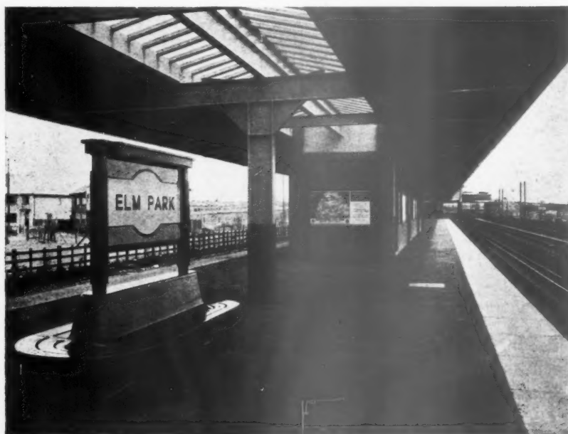
A neat example of a railway station in welded steel. See Mr. R. Moon's lecture reported here.
